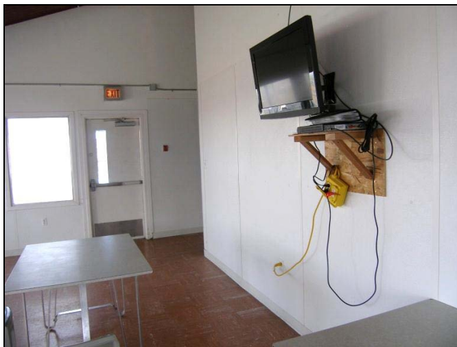
Figure 4. OIG photo of an inmate dining area with a non-detention grade exit door at the Crow facility.
