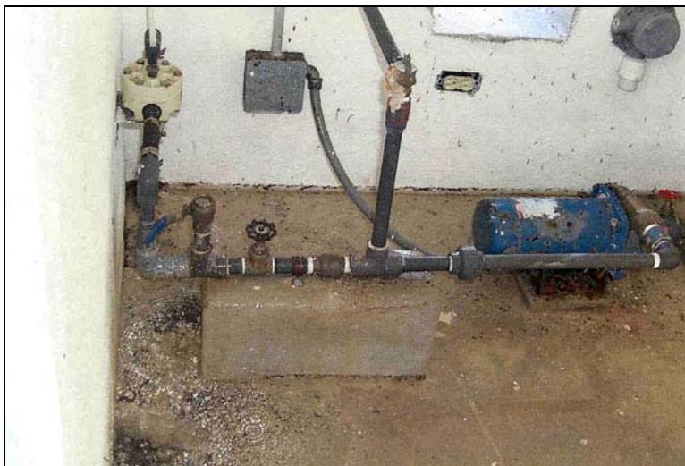
Figure 8. Barrigada Heights Station – This electrical motor was resting in standing water, causing an electrical hazard.
