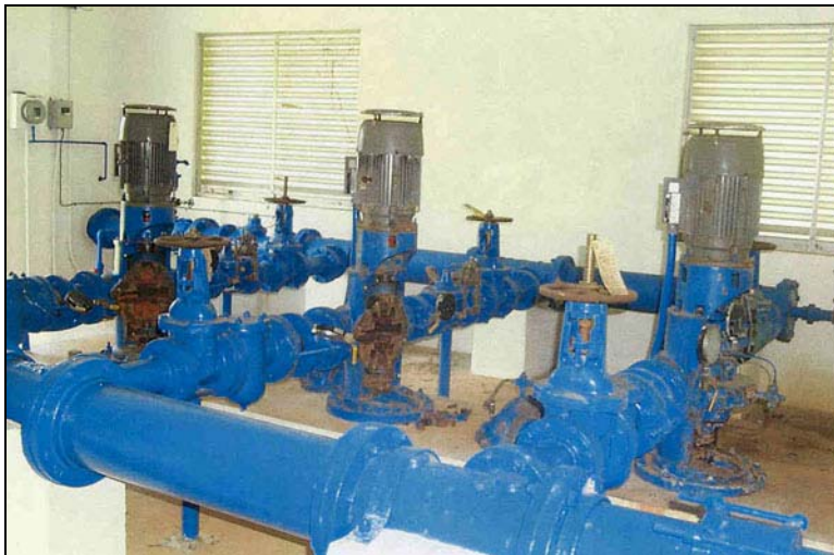
Figure 6. Asan Springs Station – The two pumps on the left were not operable because the impellers had been removed for reasons that we were unable to determine.
