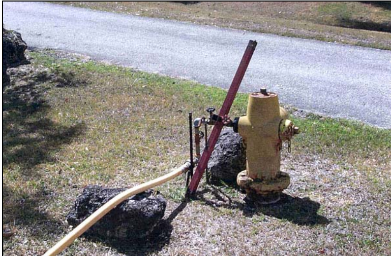
Figure 11. Illegal Hookup – A property owner had illegally tapped into this fire hydrant that was located on his property.
