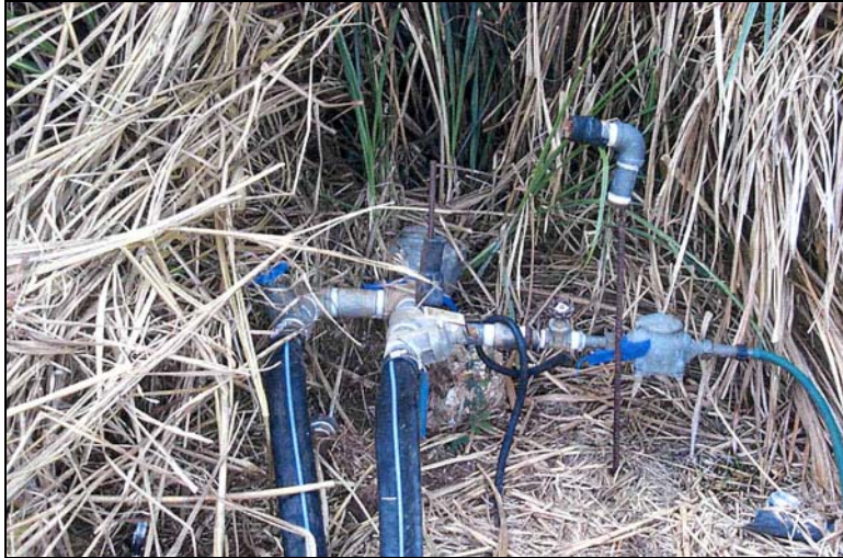
Figure 10. Illegal Hookup – Illegal hookups were made from this water meter on private property.
