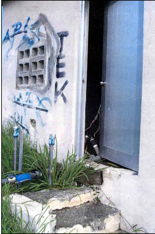
Figure 1. Old Santa Rita Station – The door to the pump room could not be closed or locked because pipes ran through the door opening.
