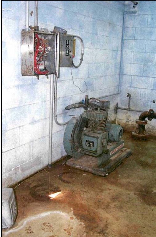
Figure 7. Sanifa Station – This pump was resting in standing water and the electrical box was unsecured.
