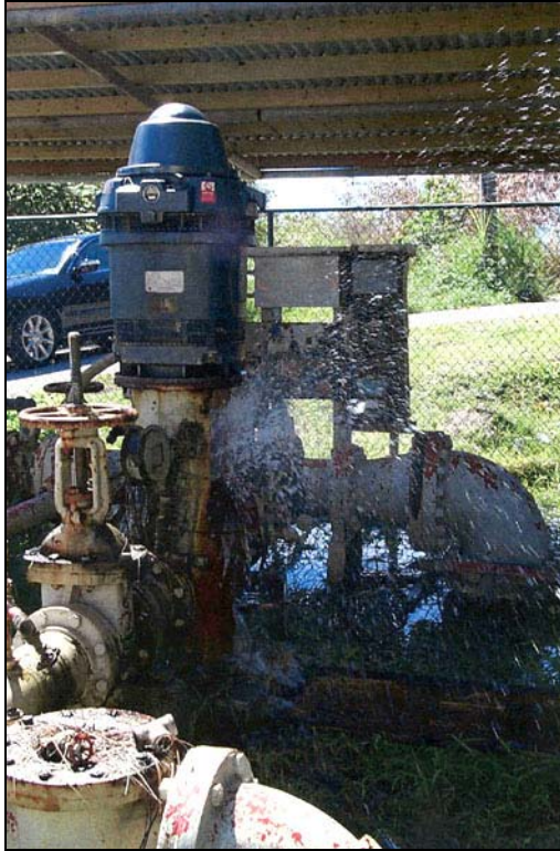
Figure 5. Barrigada Heights Station – Water gushing from outdoor pump.
