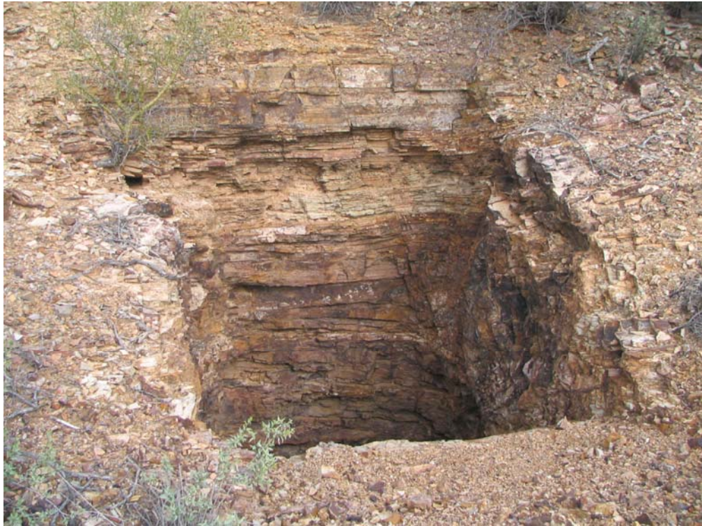
This open shaft was typical in that it was not fenced or marked. We estimated that it is approximately 60 feet deep.
