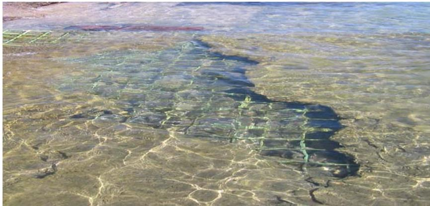
*Washouts in the new South ramp after the July 2003 concrete pour left the reinforcing steel exposed. (Photo Courtesy of the Department of Planning and Natural Resources)*
