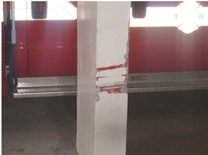
Figure 1. Damage to the structural column at the Tutu Fire Station. Also note the closeness of the fire truck to the column in the adjacent garage bay. (OIG photo)
