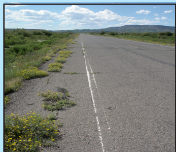
AN EXAMPLE OF A PAVED ROAD ASSESSED TO BE IN POOR CONDITION.
