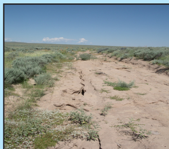
AN EXAMPLE OF AN UNIMPROVED ROAD ASSESSED TO BE IN VERY POOR CONDITION.
