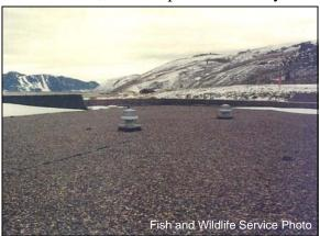
This fish production flat roof was not designed to withstand the heavy snows that occur in Wyoming. Employees continue to work in the building although a roof collapse warning was issued.
