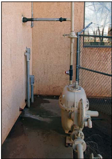
Flexible gas line components replaced the old gas lines to accommodate the shifting walls. Shifting walls could rupture gas lines, causing an explosion in the academic buildings.
