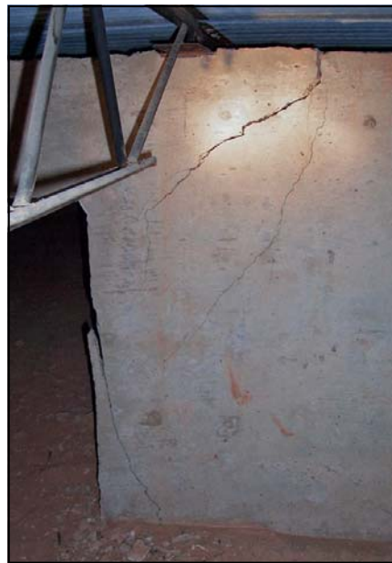
Crumbling and unstable foundations are causing school walls to shift and creating the potential for a life-threatening accident in the academic buildings.
