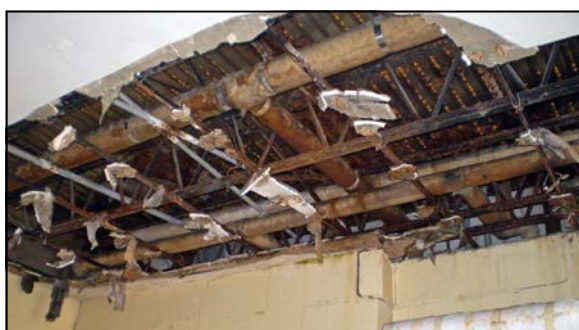
Water damaged ceiling in a condemned dormitory that is being accessed, possibly by children.
