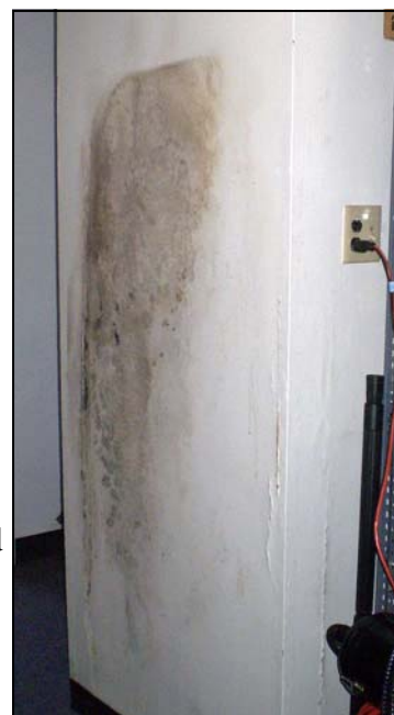
Mold in employee work area. Note: We understand that this wall has since been removed, but a mold remediation expert was not used.
