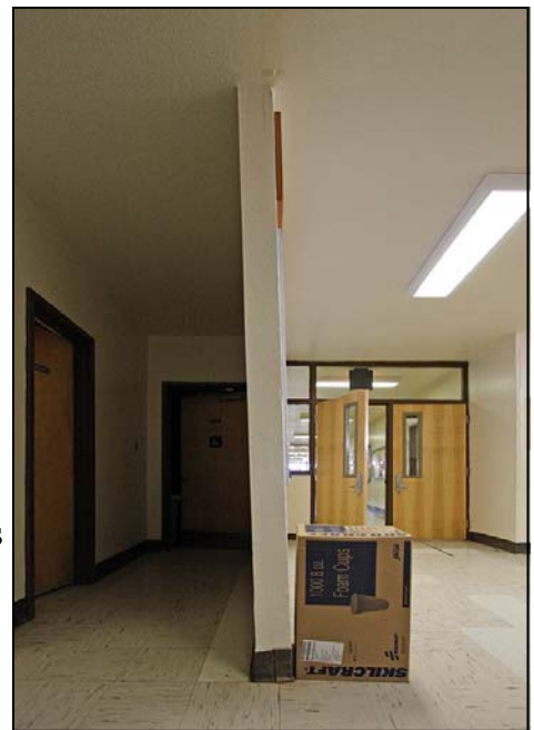
Crumbling foundations in the academic buildings at Chinle Boarding School are causing entire walls to move.
