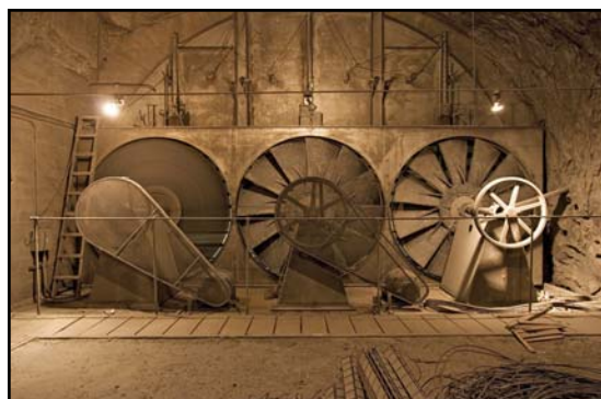
The Tunnel houses three large fans used for exhausting carbon monoxide out of the Tunnel. Two of the three fans operate, but only one at a time at low speed.
