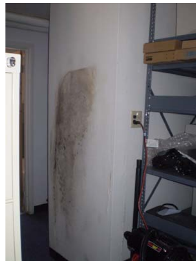
Mold in employee work area. Note: We understand that this wall has since been removed, but a mold remediation expert was not used.
