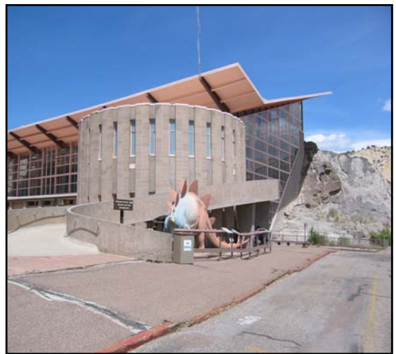
The Quarry Visitor Center incorporates the fossil rock face as one of its walls. This fossil wall will be damaged if the exhibit wall or the building collapses. NPS Photo
