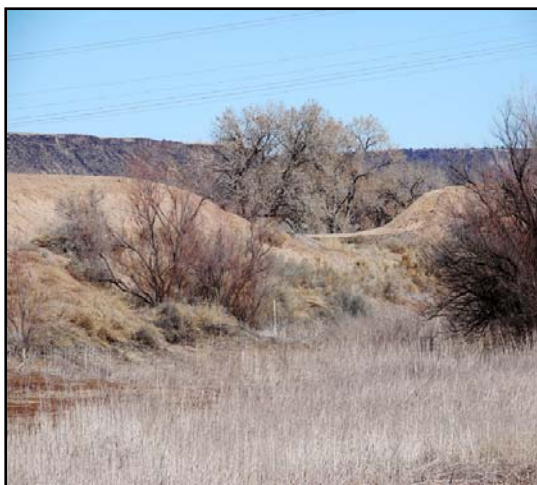
BIA partially breached the Santa Ana Dam in 1997 as a stop-gap measure to prevent a dam failure. During heavy rains, water is diverted through the breach away from populated areas.
