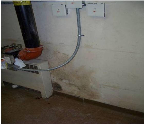
Water damage and mold in the Library OIG staff photo
