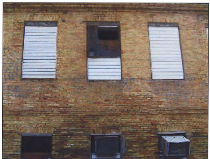
A missing air conditioner leaves an open hole in the wall of the evidence room.
