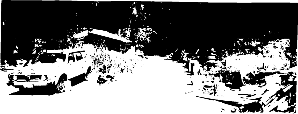
Figure 1. A ramshackle structure, surrounded by debris, on an unpatented claim in the Medford, Oregon, area. (Office of Inspector General photograph)
