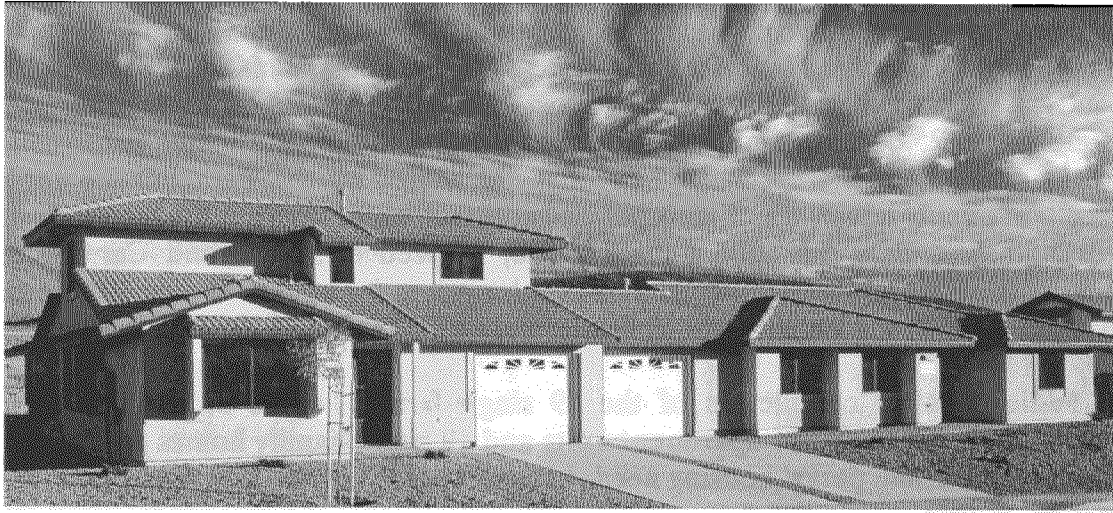
Figure 3. A duplex constructed by the U.S. Army Corps of Engineers. (Office of Inspector General photograph)
