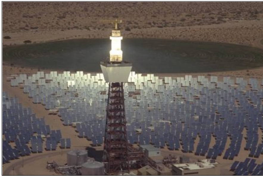
Figure 2. This is a solar project in California that uses a central power tower in the middle of a circle of mirrors. Source: BLM.
