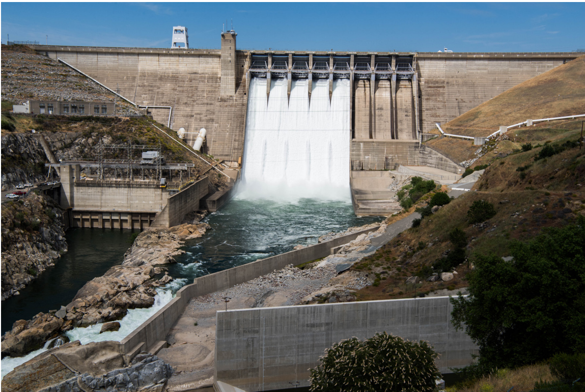
Folsom Dam, located on the American River in Sacramento, CA.
