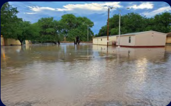
Flooding at the school in 2018.
