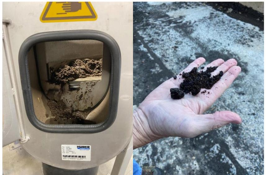
A dewatering system used to treat sludge (left) and the sludge treated to biosolid standard that results (right).
