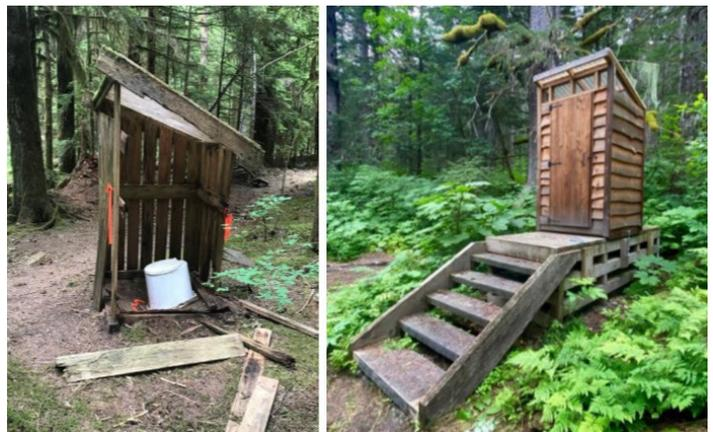
The privy on the left would be banned under the EPA's definition of a large-capacity cesspool if used by more than 20 people per day. The privy on the right would not be banned based on its design and unique way of treating waste.
