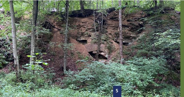
Highwall and collapsed entrances in Morgantown, WV. This site includes approximately 4,725 linear feet of highwall ranging in height from 15 to 40 feet, 13 open entrances, at least 10 collapsed entrances, and approximately 2,100 feet of clogged stream.
