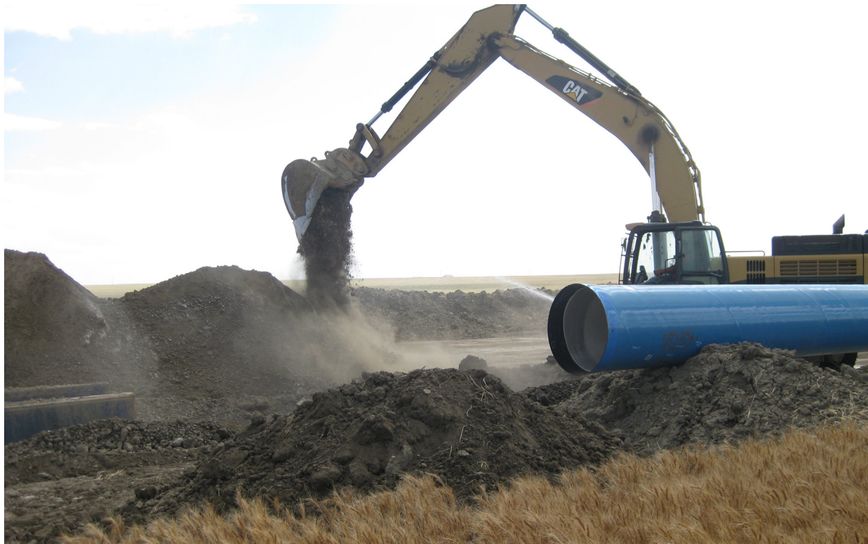
Construction on the Rocky Boy's/North Central Montana Regional Water System.
