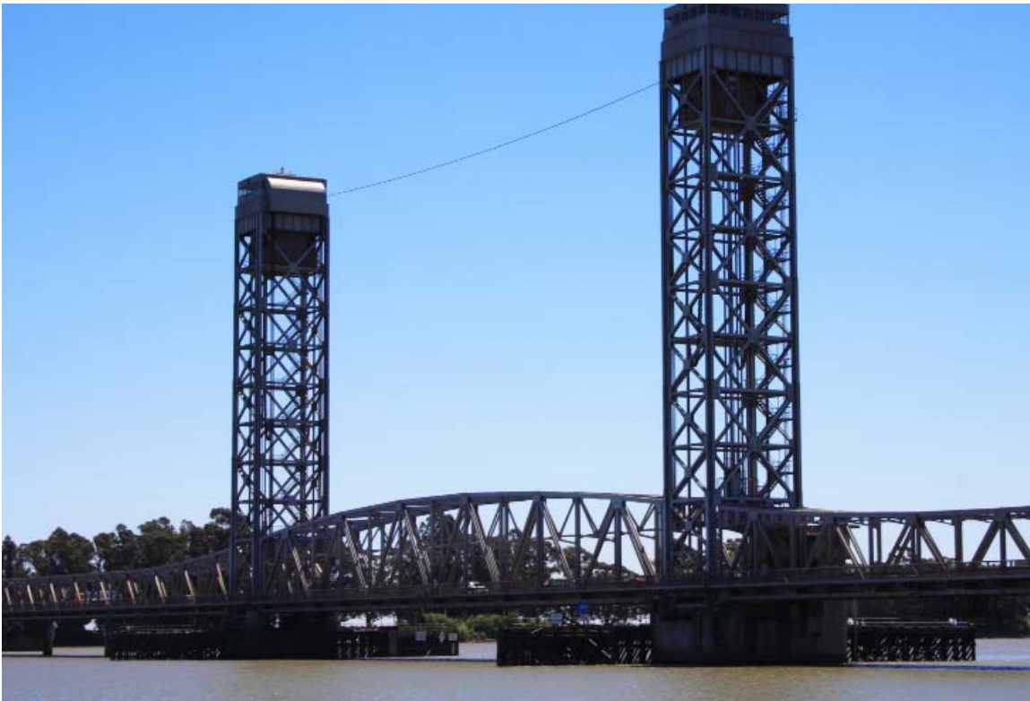
The Helen Madere Memorial Bridge spans the Sacramento River, which contributes to the Bay-Delta water supply.
