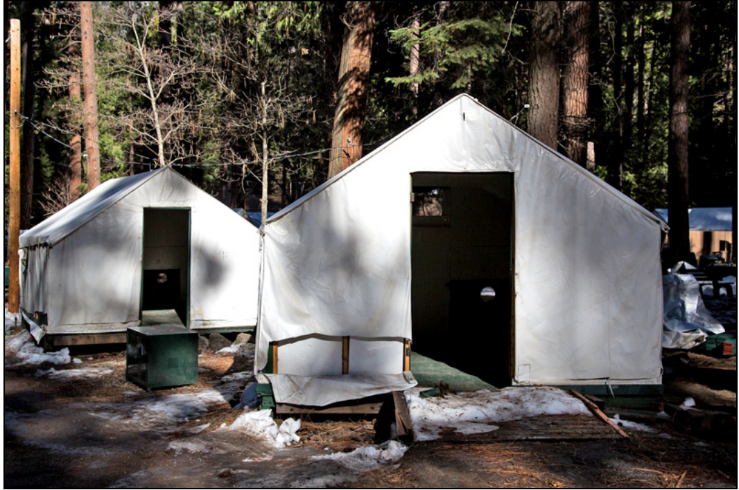
Figure 1. Signature tent cabins in Curry Village that are in the process of being deconstructed. The canvas has been cut away to show the foam insulation in the walls. Source: OIG team photo.
