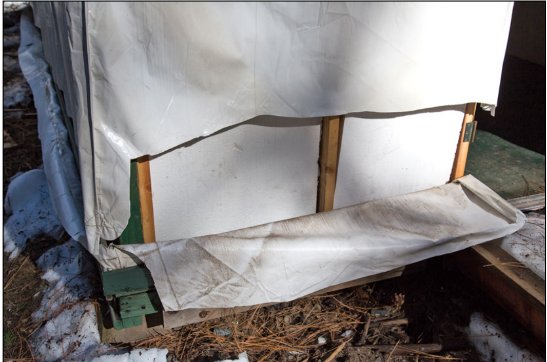
Figure 2. A close-up of the foam insulation in the walls of the Signature tent cabins. Source: OIG team photo.
