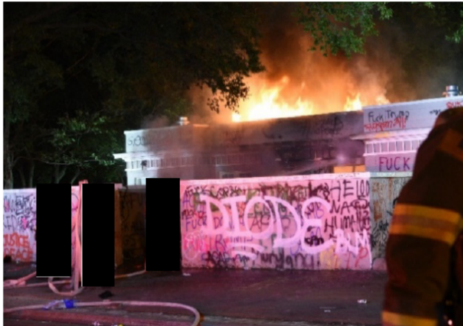
Figure 3: Fire at Lafayette Park Comfort Station on May 31, 2020
